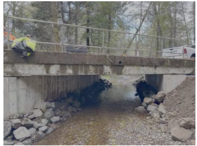
New bridge on Sutton Creek
