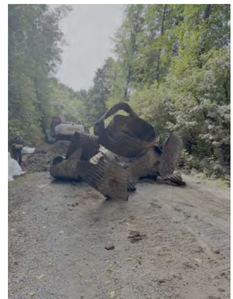
Upper Culvert removed
